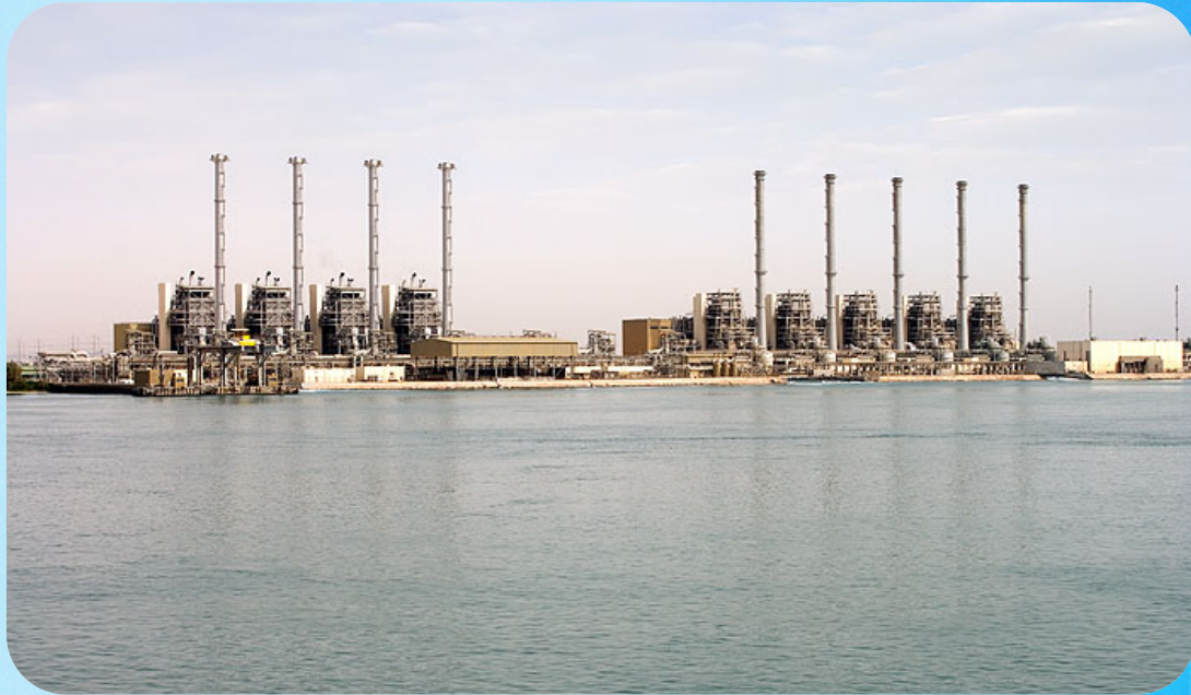
Azzia desalination plant, Saudi Arabia
