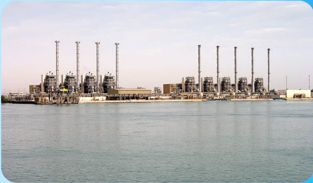
Azzia desalination plant, Saudi Arabia
